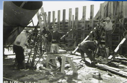
Photo No. 30. Drilling curtain holes through concrete at Elevation 188 in monolith 19. View downstream. Neg. No. CD 6186 2-4-65 (Courtesy of California Department of Water Resources)
