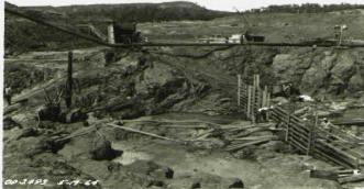
(Courtesy of California Department of Water Resources)
